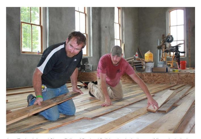
Jerry Taylor, left, and Shane Fuller of Penland Builders begin the layout of floor planks in the courtroom of the Historic Courthouse. To prevent damage to the boards during the renovation, each plank was removed and placed in storage. The boards were then carefully planed to restore much of their original color and patina and are now ready for service of another 140 years.
